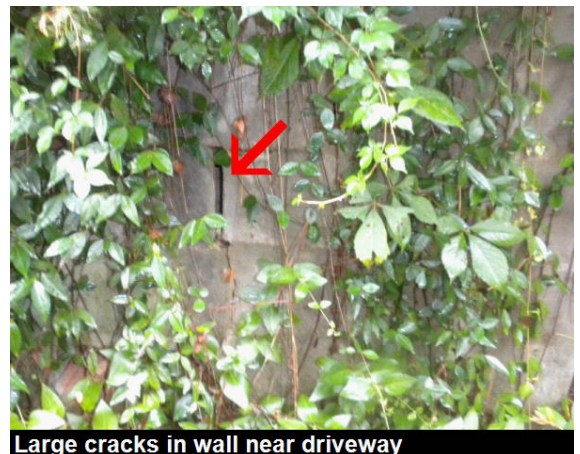
Large cracks in wall near driveway
