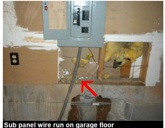
Sub panel wire run on garage floor
