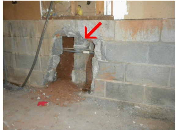
Damage to block wall under panel
