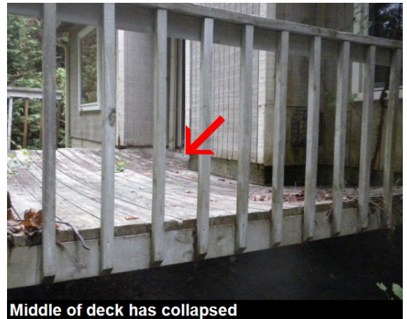
Middle of deck has collapsed
