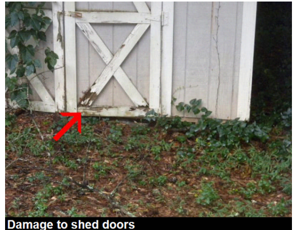
Damage to shed doors
