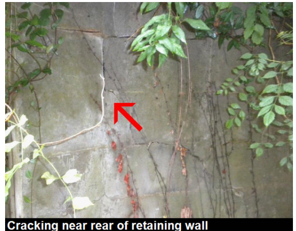
Cracking near rear of retaining wall
