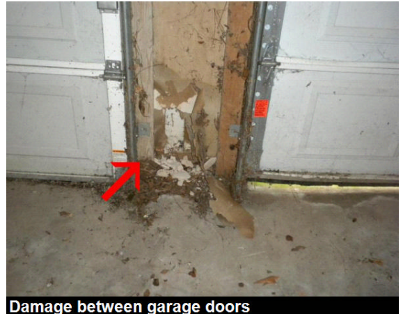
Damage between garage doors
