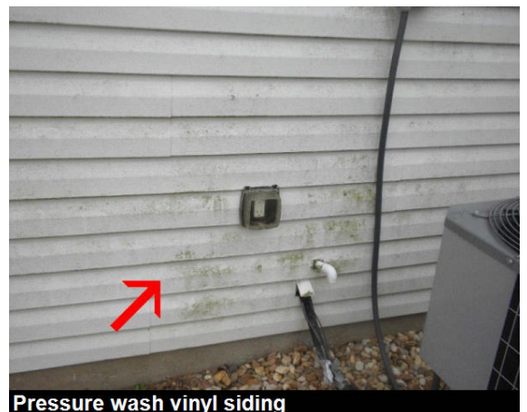
Damaged vinyl siding @ rear
