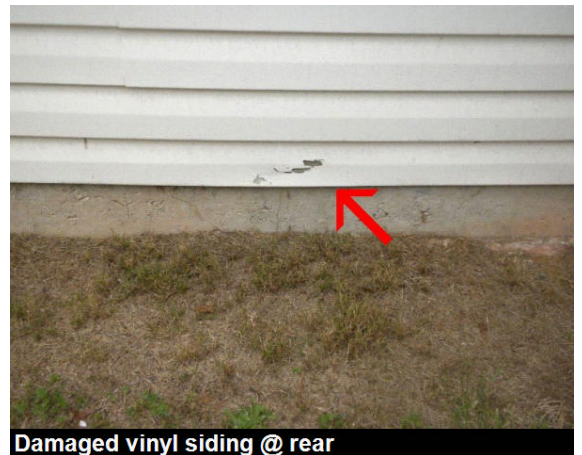
Damaged vinyl siding @ rear
