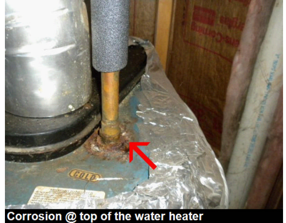
Corrosion @ top of the water heater
