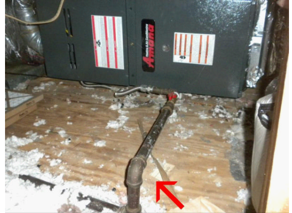
No drip leg on the gas line
