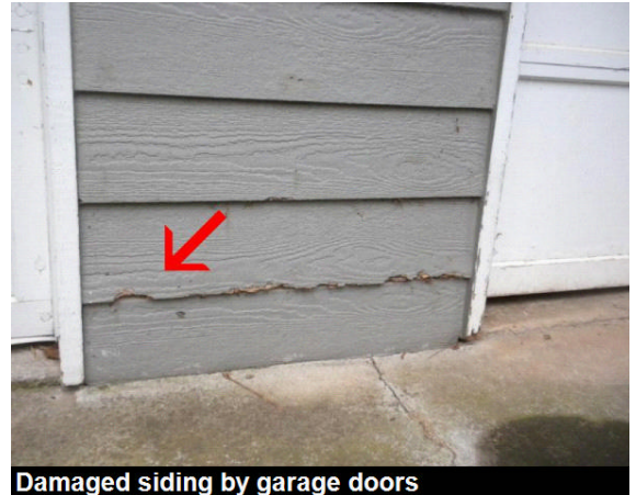
Damaged siding by garage doors
