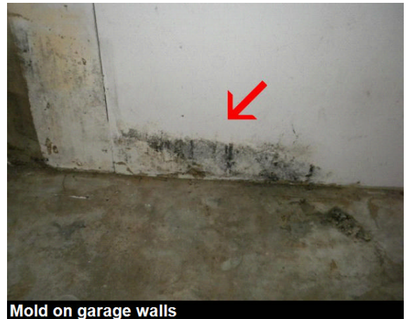
Mold on garage walls
