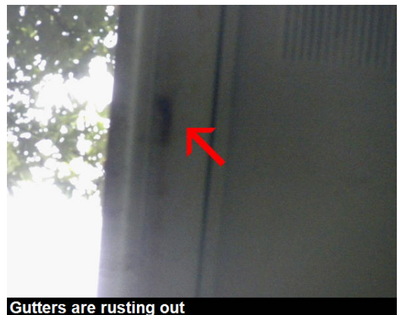
Gutters are rusting out
