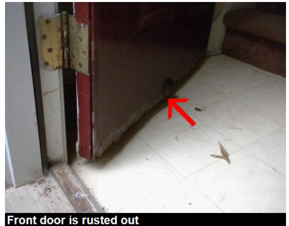
Front door is rusted out
