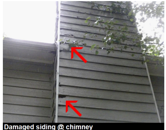
Damaged siding @ chimney
