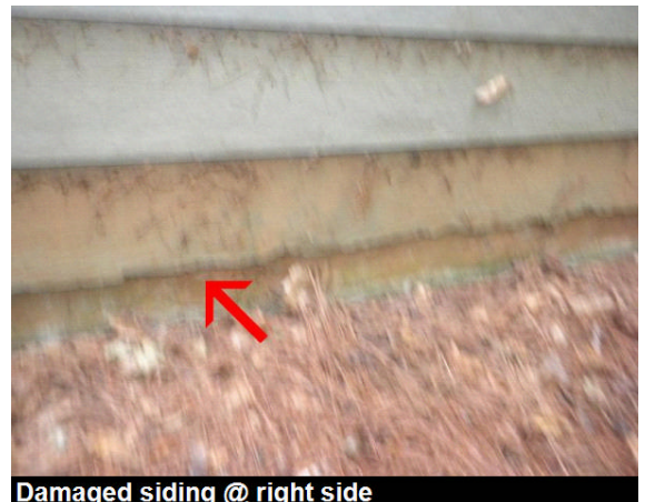
Damaged siding @ right side
