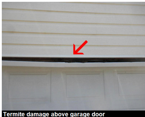
Termite damage above garage door
