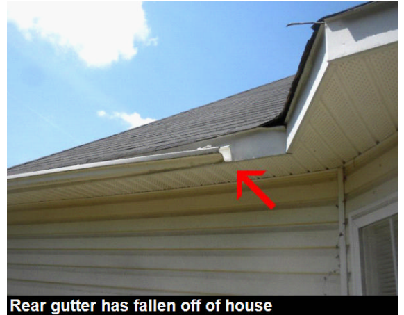
Rear gutter has fallen off of house
