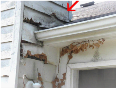
Damage @ chimney chase
