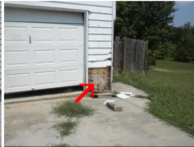
Missing siding @ right
