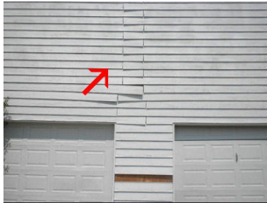
Damaged siding @ right
