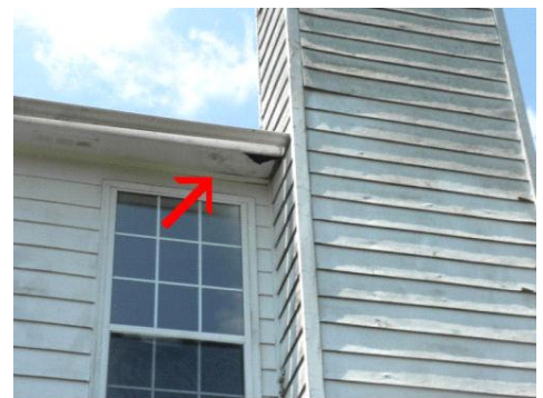
Damaged soffit @ rear
