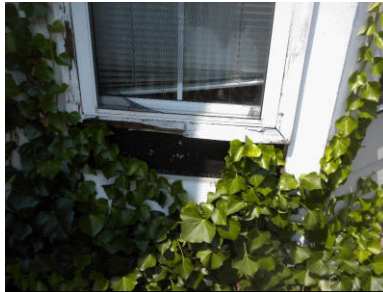
Missing siding @ front
