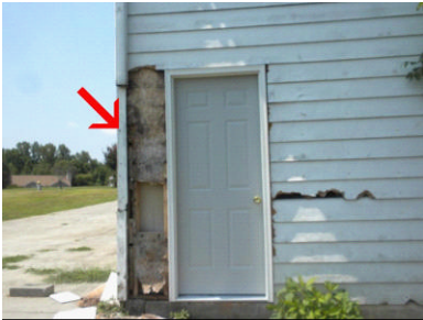
Missing siding @ garage
