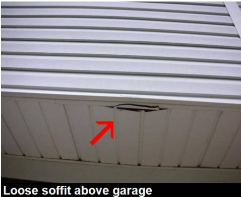
Loose soffit @ right side
