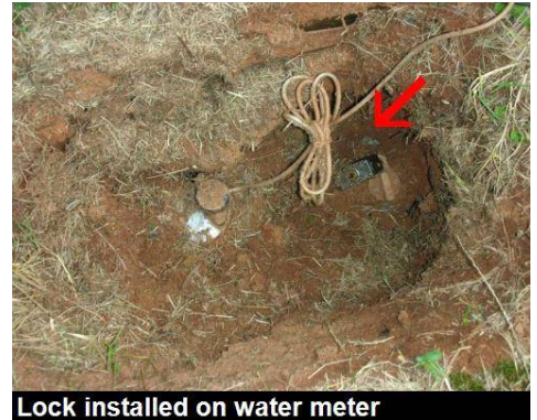
Lock installed on water meter
